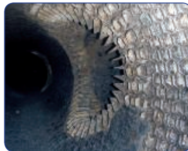
A refractory repair involving Hexmesh, hex cells, and variable tabs
