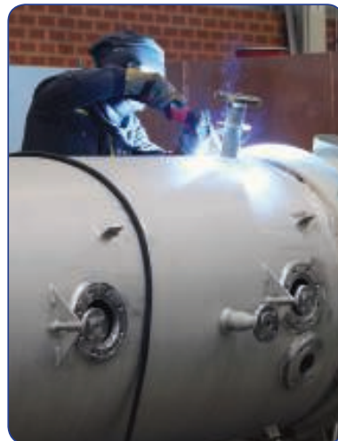
One of the two columns under construction in BUTTING's Knesebeck facility
