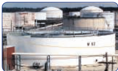
Concentric tanks help to minimize the footprint of the OXIGEST system
